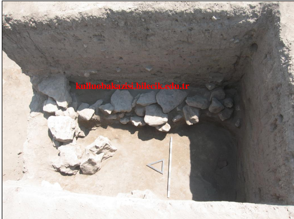
Figure 7. Trench AB 17. The stone foundations of the building dated to the Transitional Period into the MBA.
