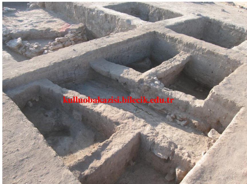
Figure 9. The walls of the period transitional to the MBA, with the EBA fortifications appearing at the upper left (from the north)
