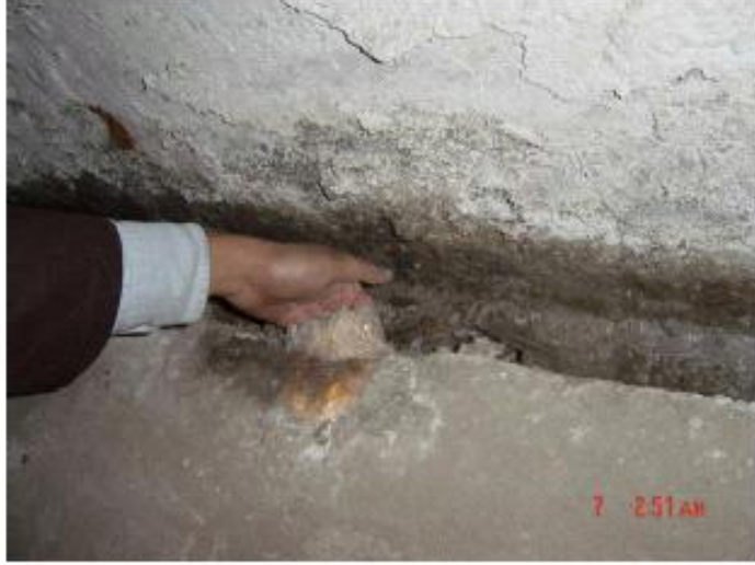
Fig. 4. Deterioration in the tunnel drainage channels.
