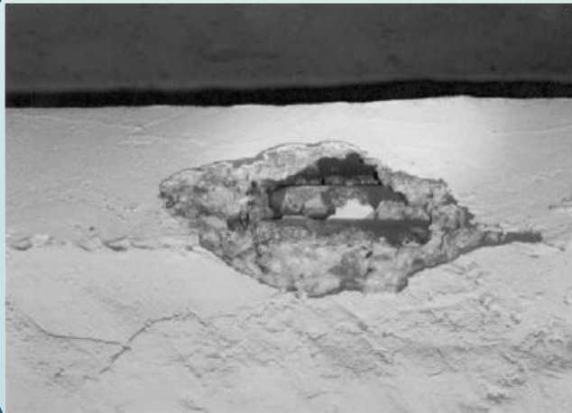
Fig. 4. Deterioration in the tunnel drainage channels.
